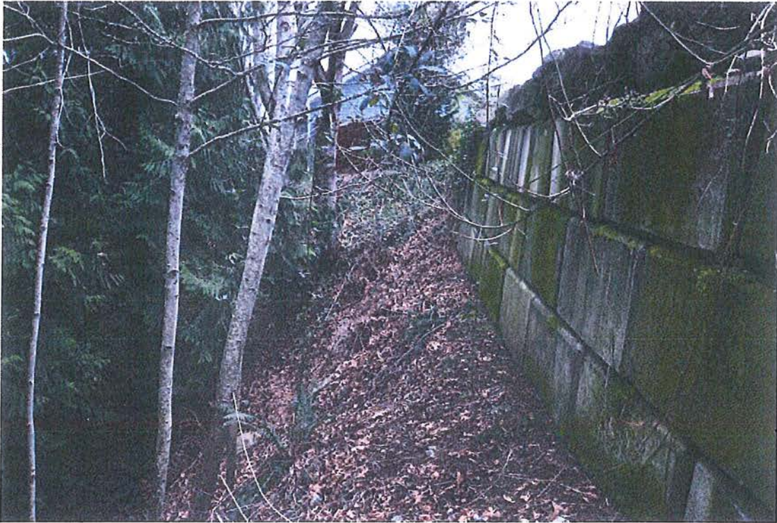
Figure 7: Retaining wall for adjacent land development along the 'top of bank' of Darough Creek.
